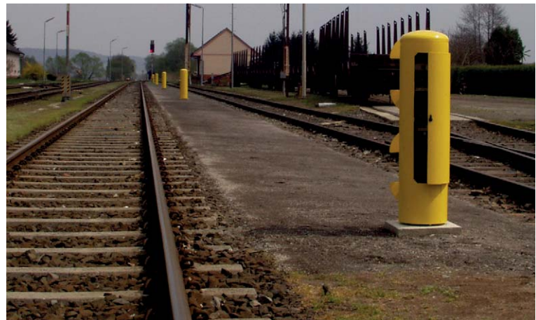
Power supply - Energy supply
