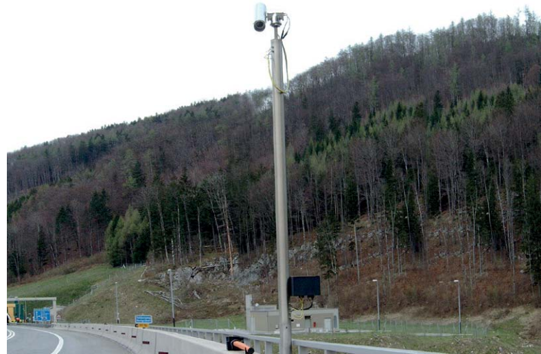
Video junction boxes
