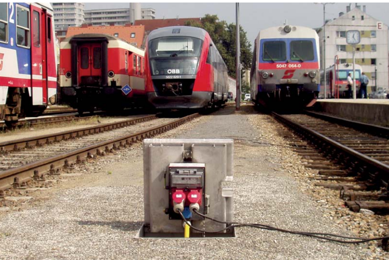
Power supply - Underground distributor
