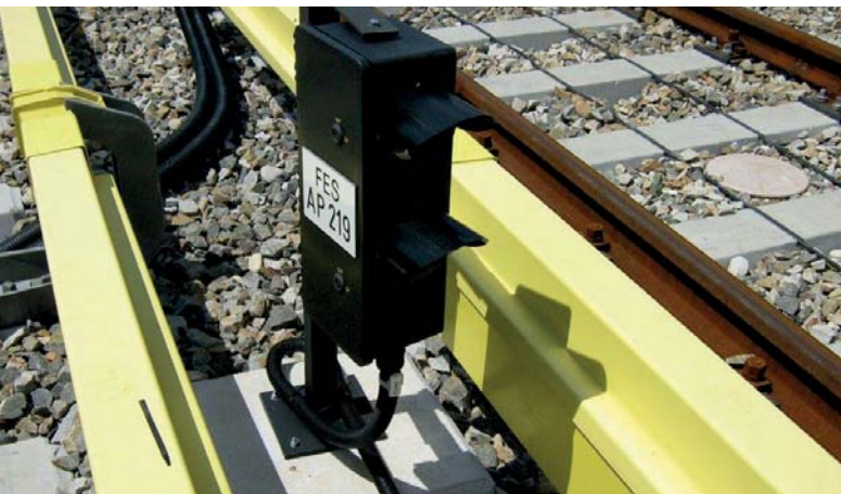
Railway LED - Light signal
