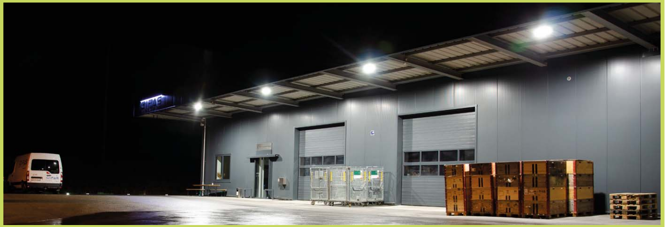
AlphaLUXX - lighting of warehouses / storage areas
