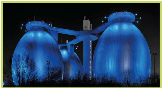
DeltaLUXX Blue - Outdoor sewage treatment plant lighting
