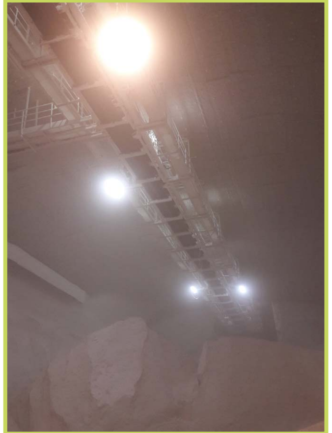
DeltaLUXX 2 HT - Lighting salt works
