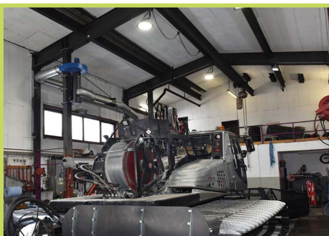
DeltaLUXX - Snow grooming workshop lighting
