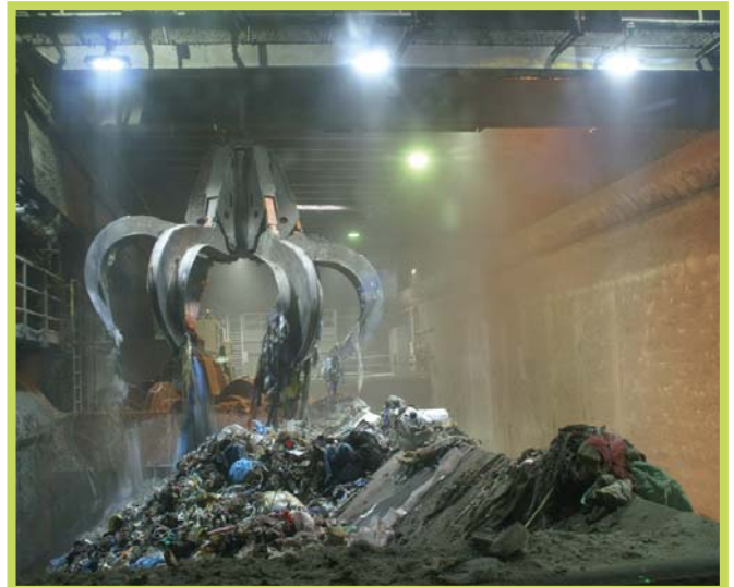
PLAZA - Lighting in waste incineration plant
