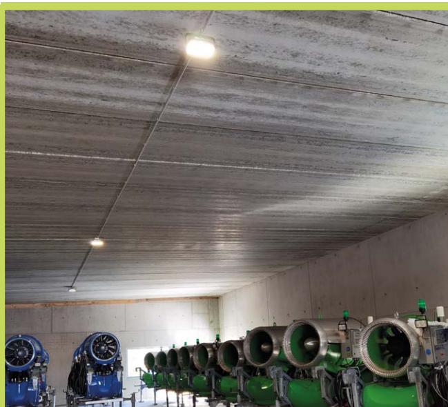
AlphaLUXX - Lighting in the power plant
