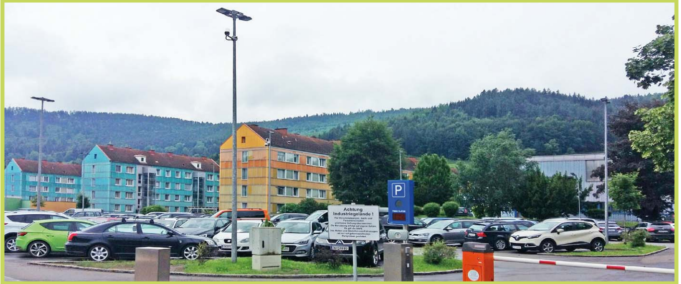
PLAZA FlatLED - Parking lot lighting
