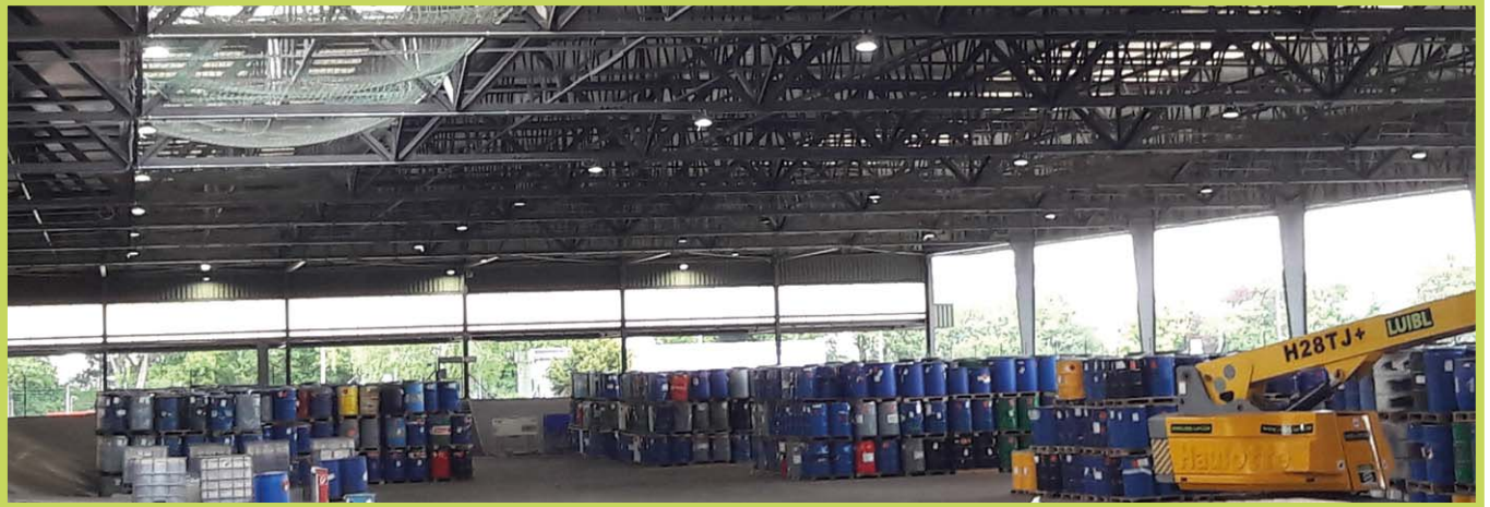
DeltaLUXX - Storage space lighting
