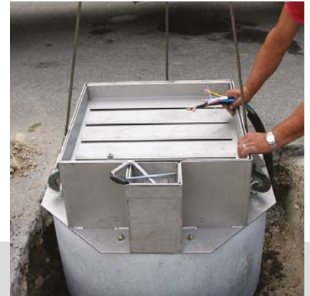
Dropping down of complete unit into the prepared casting pit with suitable lifting aid (crane).
