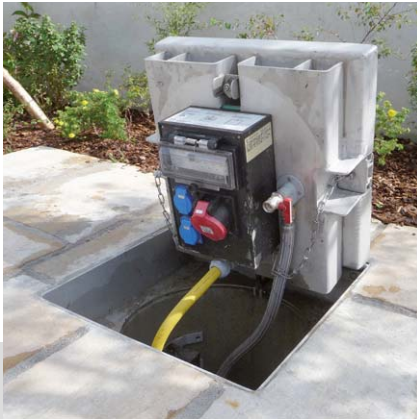
Market town of Schneegattern: Under-ground energy system PIAZZA 540 with two cable outlets and water connections.
