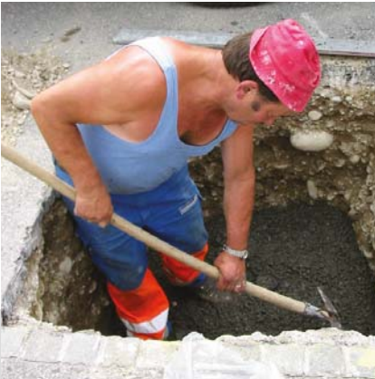
Drawing out of casting pit on the basis of the required dimensions. Installation of a proper foundation as well as a drainage system.
