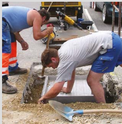
Filling of unit used, and producing a concrete sleeve over all of the stainless steel construction (see technical drawing).
