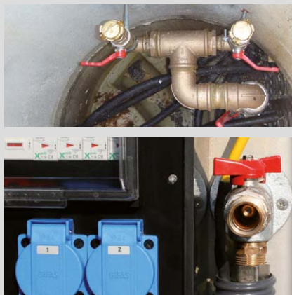
Water supply in / on the shaft or water connection at the shaft cover.
