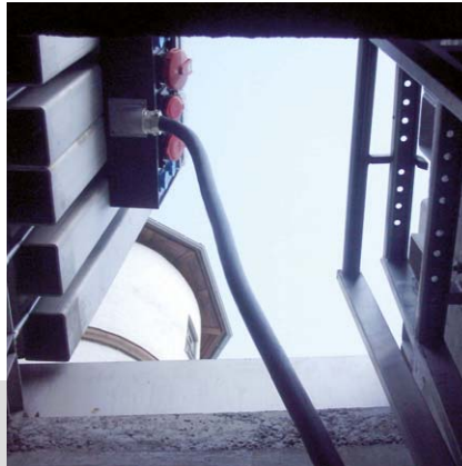
Junkers-Schlössle Götzis: Under-ground distributor PIAZZA 1000 for power supply as well as a manhole.
