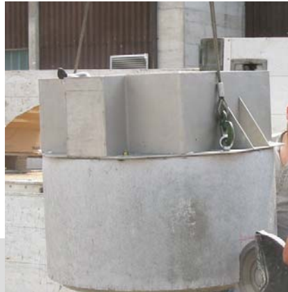
The stainless steel construction, mounted onto the concrete ring, is prepared for installation. Openings for supply cables need to be cut out of the concrete ring.
