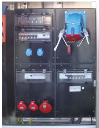
Stainless steel distributors for shipping piers Verbund power plant Abwinden-Asten
