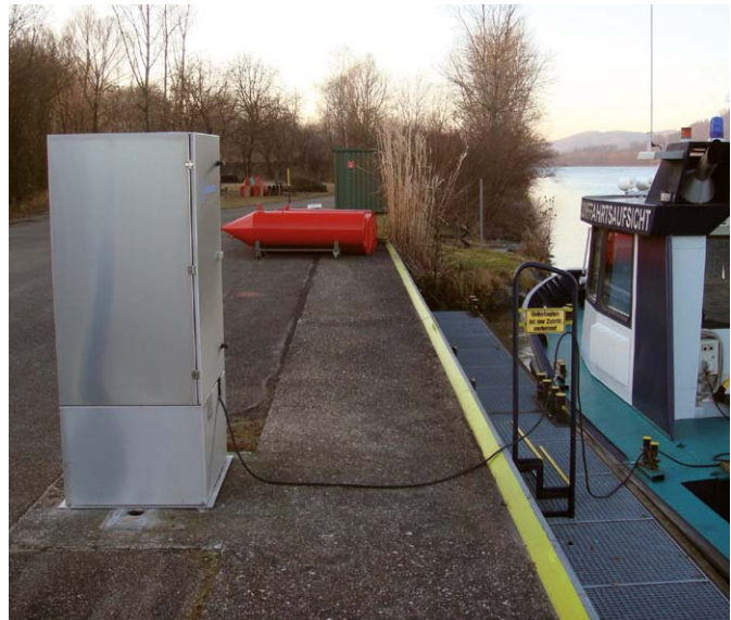
Stainless steel socket distributor - TIWAG Jenbach
