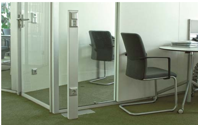
GAS 100 - Office building Borealis Innovation Headquarters Linz
