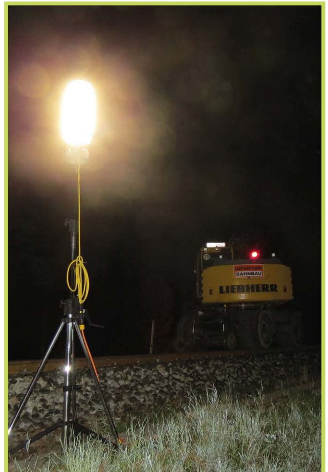
ApolloLED - Construction site use
