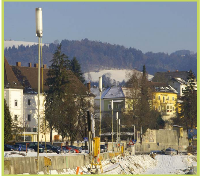
ApolloLED - Lighting on construction sites
