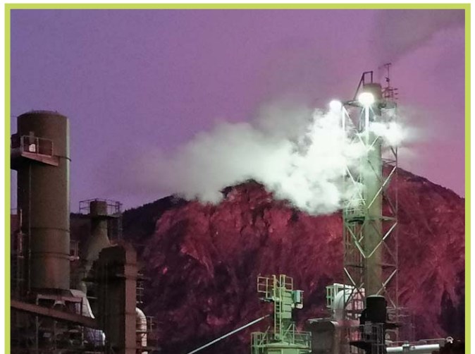
High Power LED - Illumination of factory premises
