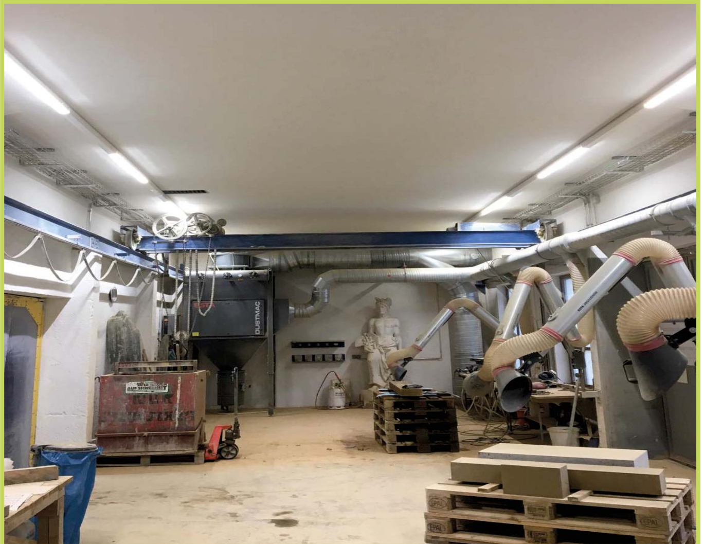
Industry Track LED - Workshop / workplace lighting
