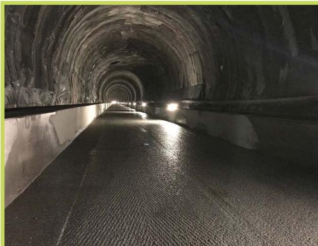
StreamLED Power - Tunnel lighting
