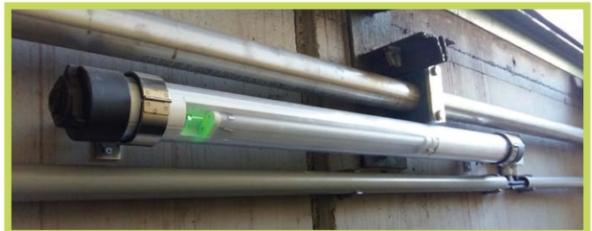
StreamLED 70 Notlicht - Emergency lighting of an energy channel
