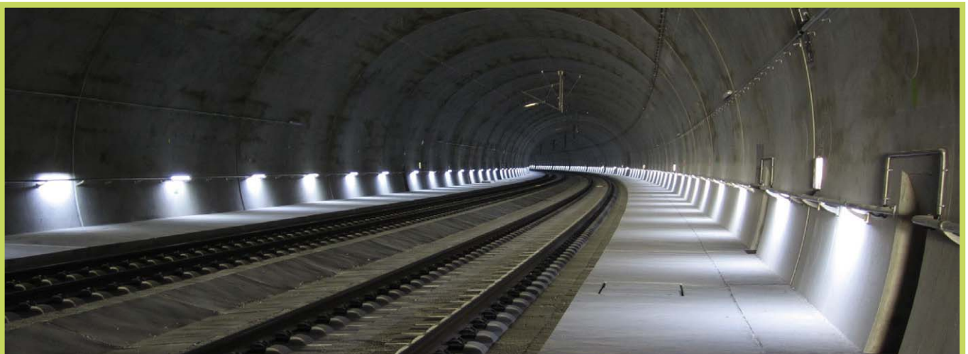
AmbitLED - Lighting the railway tunnel
