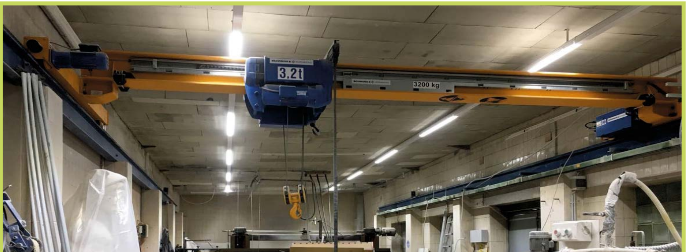
Industry Track LED - Workshop lighting
