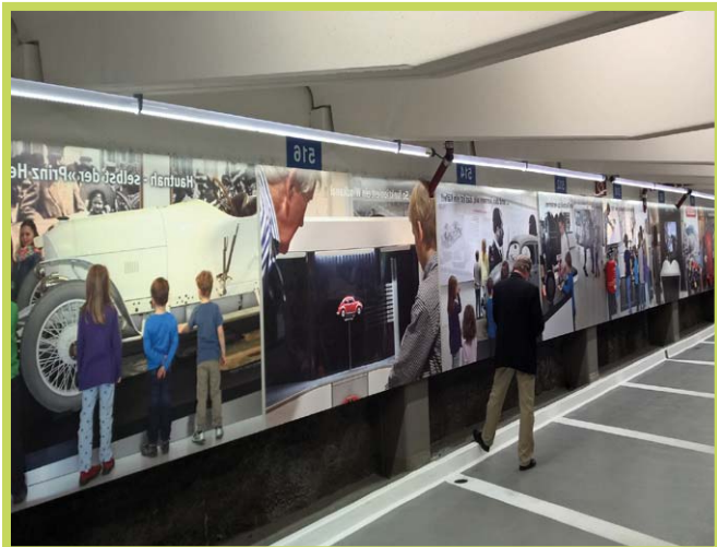
StreamLED Power - Underground parking garage lighting
