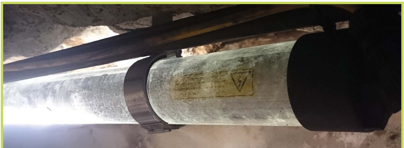
StreamLED Power - Stollenbeleuchtung
