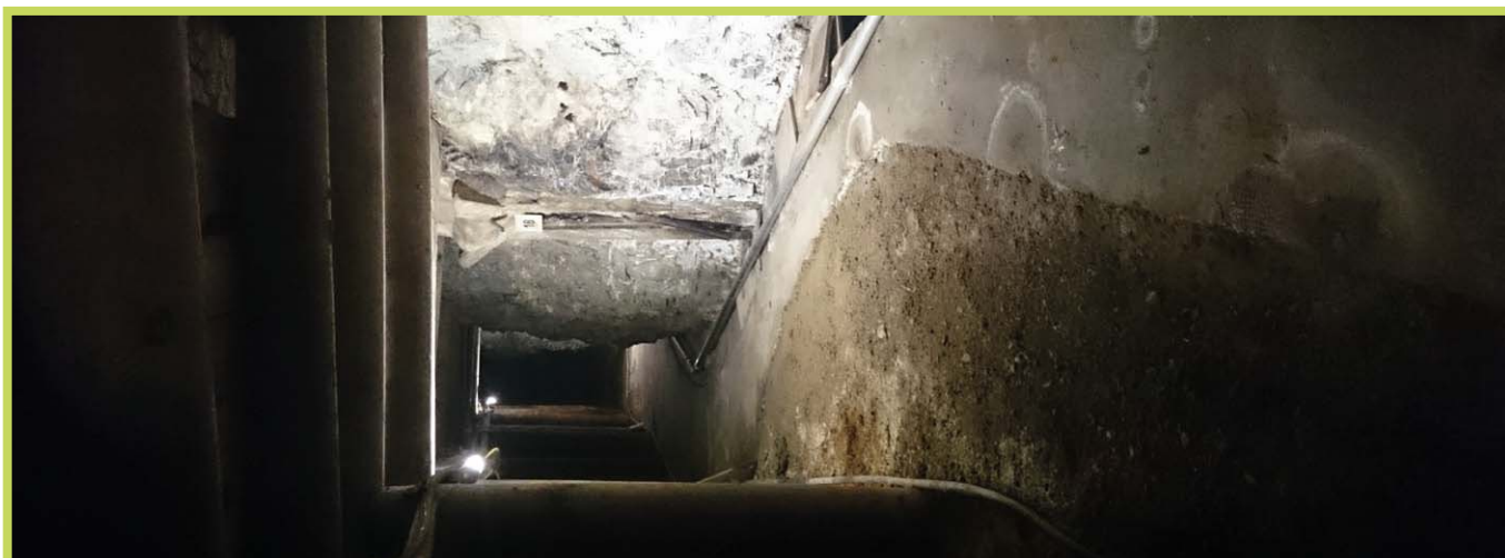
StreamLED Power - Stollenbeleuchtung
