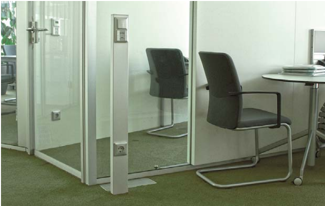
GAS 100 - Office building Borealis Innovation Headquarters Linz
