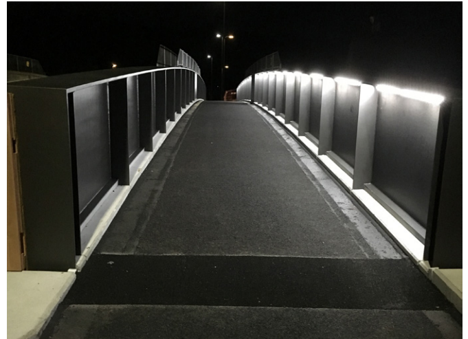
Pedestrian bridge Brügg
